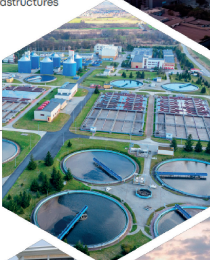
Water Treatment Infrastructures
